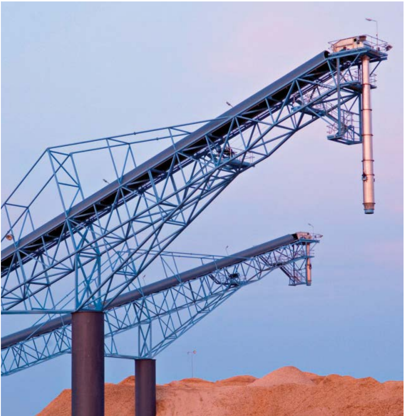
Plantation hardwood stockpile conveyors at Midway's Geelong facility
